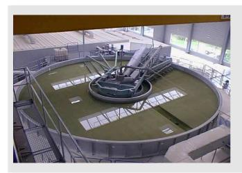
Example for a flotation plant (paper mill)
