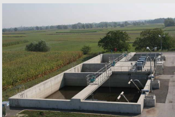
Wastewater Treatment Plant of the Croatian Town Virje (5,000 p.e.) operating with two SB-reactors, completely designed and equipped by Biogest International GmbH.
