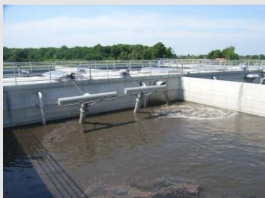
The maintenance-free BSK®-decanter is installed in plenty of SB-reactors with utmost success.
