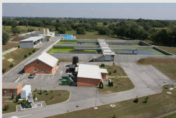
Bird-eyes view of the wastewater treatment plant being designed and realized by Biogest International GmbH for the Croatian town Koprivnica (100,000 p.e.) – operating according to the SBR-process (4 reactors).
