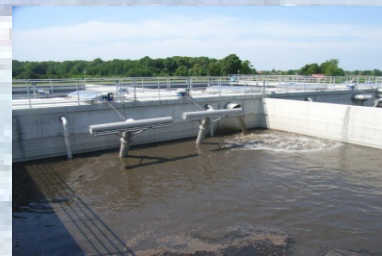
BSK ® -Decanters for the Croatian-WWTP Koprivnica
