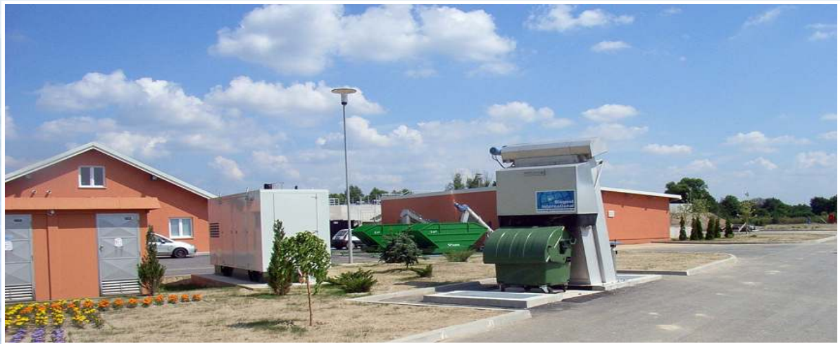
An automatic coarse screen ensures that coarse material like limbs, tins, cadaver, etc. is discharged.
