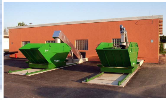
Dropping of sand and solids out of the pre-treatment station. By use of a special washing method, the majority of organic ingredients are led back to the wastewater.
