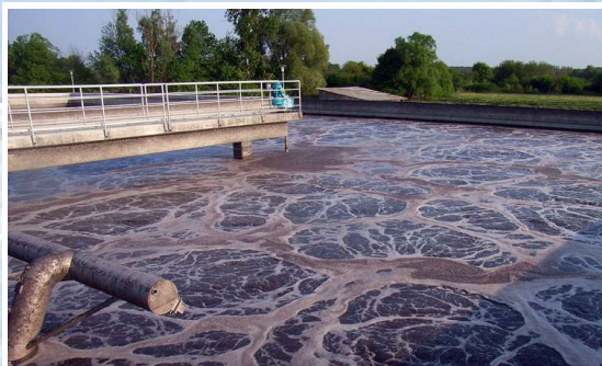
View of one of the four SB-Reactors with central placed HyperClassic-Stirrer and BSK®-Decanter to extract clear water.
