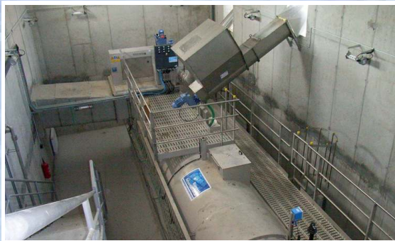
Compact pre-treatment station for pre-treatment of wastewater (fine screen, aerated sand and grease trap). For separation of sand, the patented "Walzensandfang" was used.
