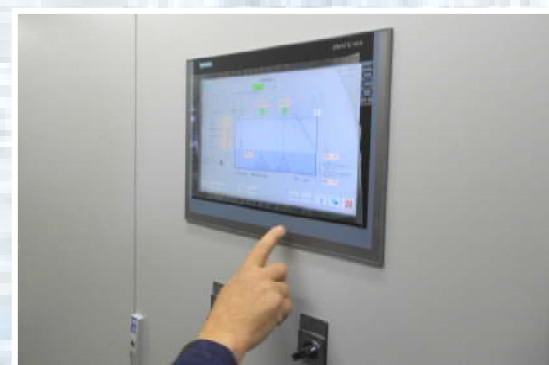
Next to the SCADA-system all data can be read by a state-of-the-art touch panel.
