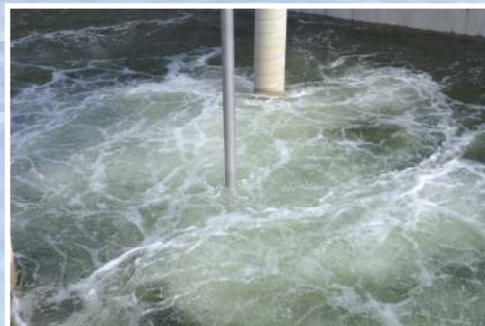
By especially developed HyperClassic®-mixing and aeration systems, the compressed air is smashed into finest air-bubbles
