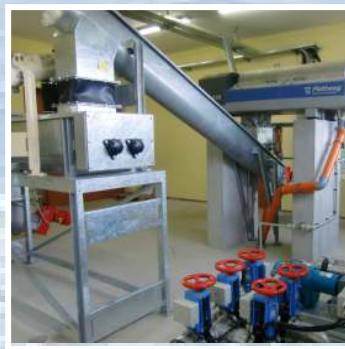
By use of rotary piston pumps the thickened sludge is discharged from the sludge reactors into the dewatering unit. Firstly, it is mixed with a polymer-solution and afterwards it is dewatered to a DS-concentration of up to 25 % in a dewatering centrifuge. Then, lime is added, which could increase the DS-concentration to up to 50 %.
