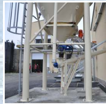
By use of rotary piston pumps the thickened sludge is discharged from the sludge reactors into the dewatering unit. Firstly, it is mixed with a polymer-solution and afterwards it is dewatered to a DS-concentration of up to 25 % in a dewatering centrifuge. Then, lime is added, which could increase the DS-concentration to up to 50 %.
