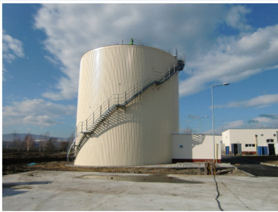
Sludge digester for anaerobic treatment of biological excess sludge and primary sludge for production of methane gas
