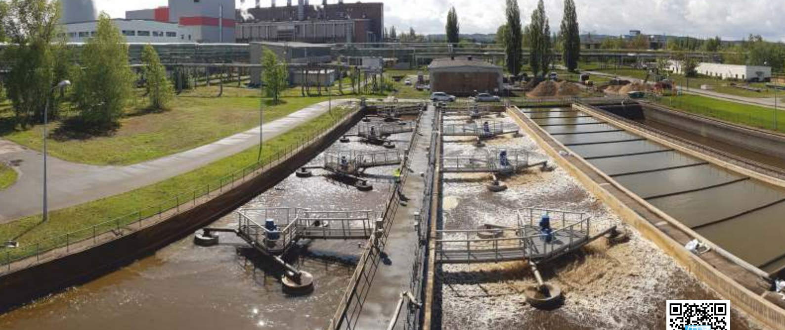
Floating BSK®-Turbines Ø 1,600 mm installed in a German industrial wastewater treatment plant
