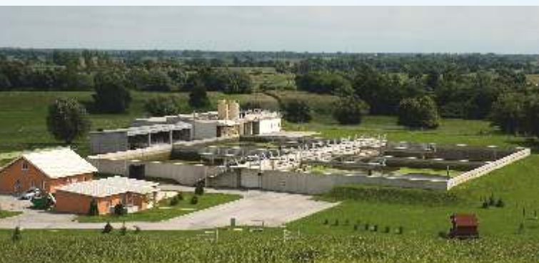
SBR-WWTP of the city of Koprivnica (100,000 p. e.)
