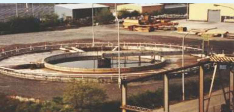
WWTP of the Adam Opel AG (Germany)
