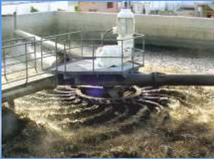
BSK®-Turbines (Surface Aerators)
