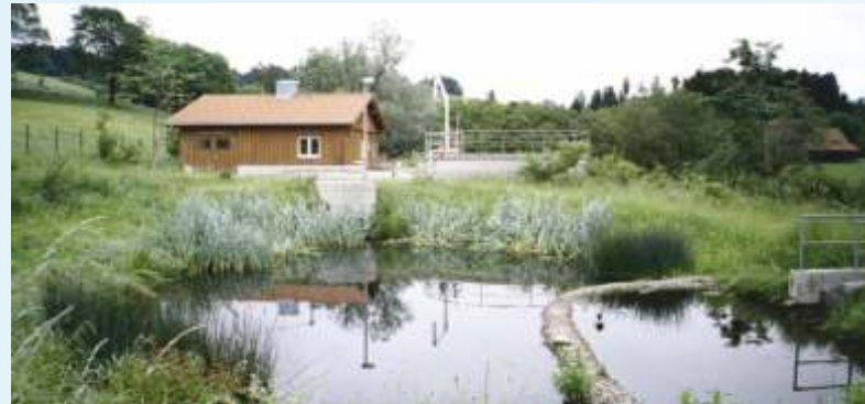
WWTP of Ebratshofen (Germany)
