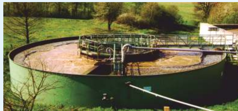
WWTP of the rendering plant Detmold (Germany)
