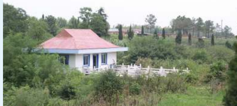
SBR-WWTP of Sopo (China)
