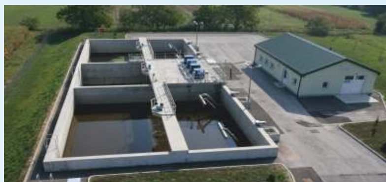
SBR-WWTP of the village Virje (Croatia)
