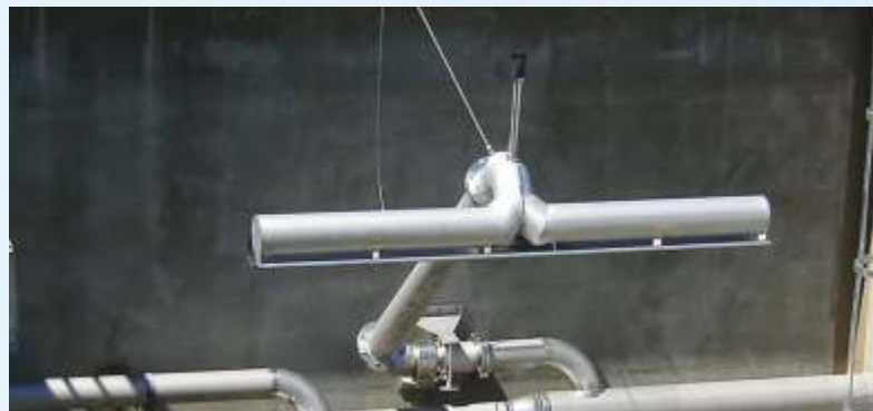
BSK®-Decanter of the WWTP Rumenka (Serbia)
