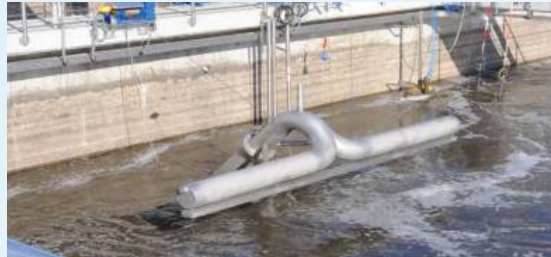
BSK®-Decanter of the WWTP Durdevac (Croatia)
