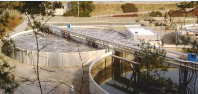
SBR-WWTP of the city of Amreya (Egypt)
