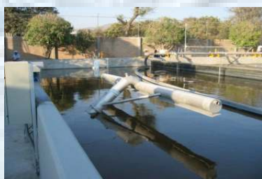
BSK®-Decanter for discharge of clear water installed at a WWTP in Mexico
